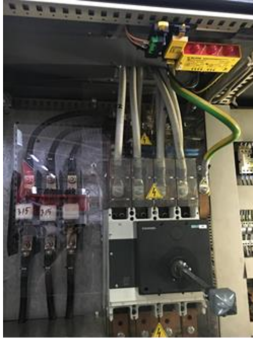
Cables from the electric panel to the injection moulding line
