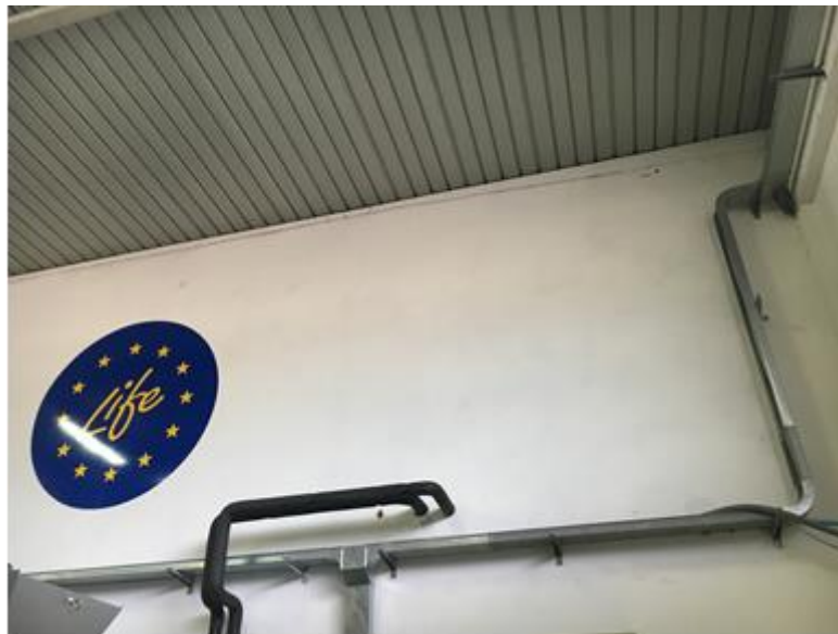
Cables connected in the electric panel
