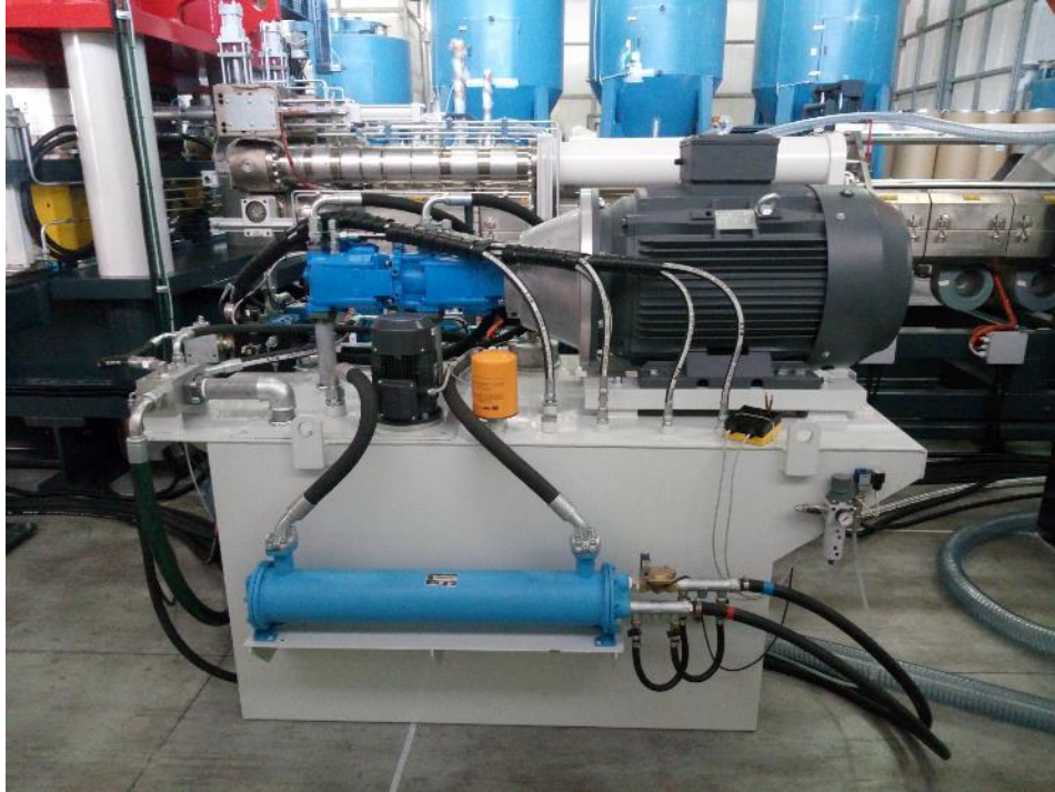
Installation of the hydraulic unit at the demonstration site
