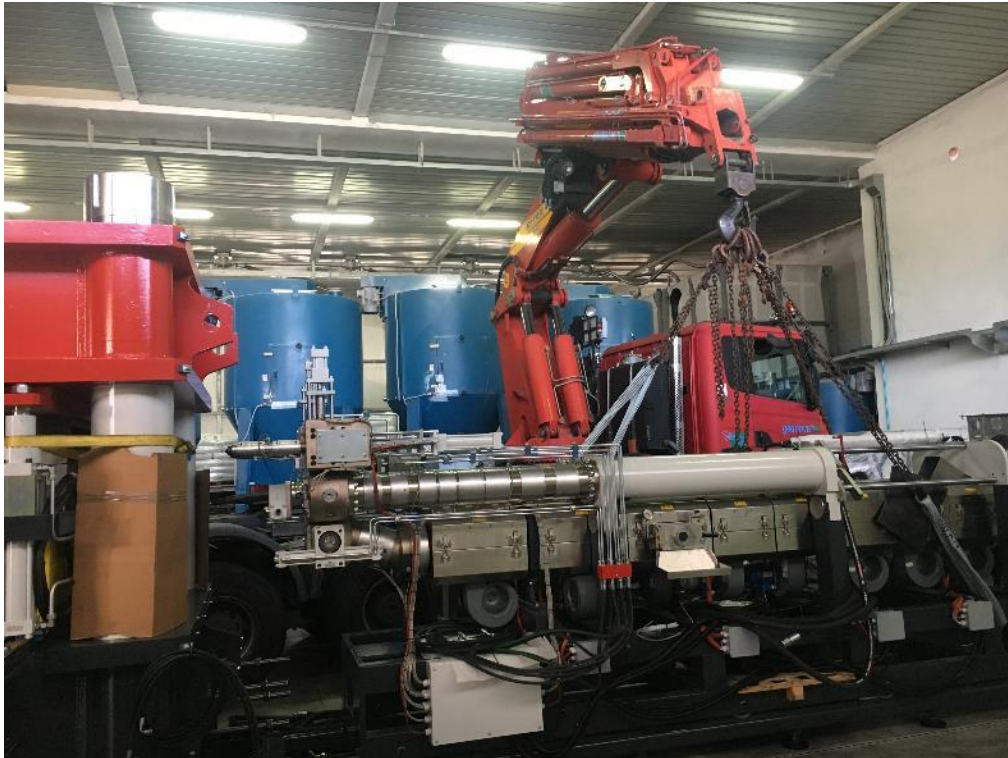
Installation of the injection unit at the demonstration site
