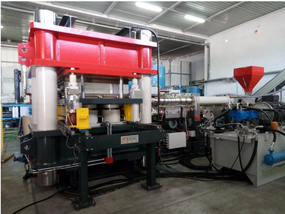
Press and mould holder installed at the demonstration site
