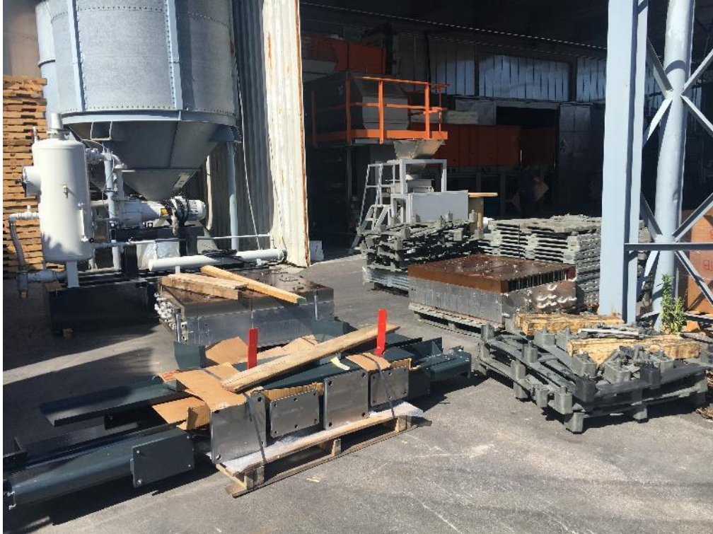
Materials and components unloaded at Selene
