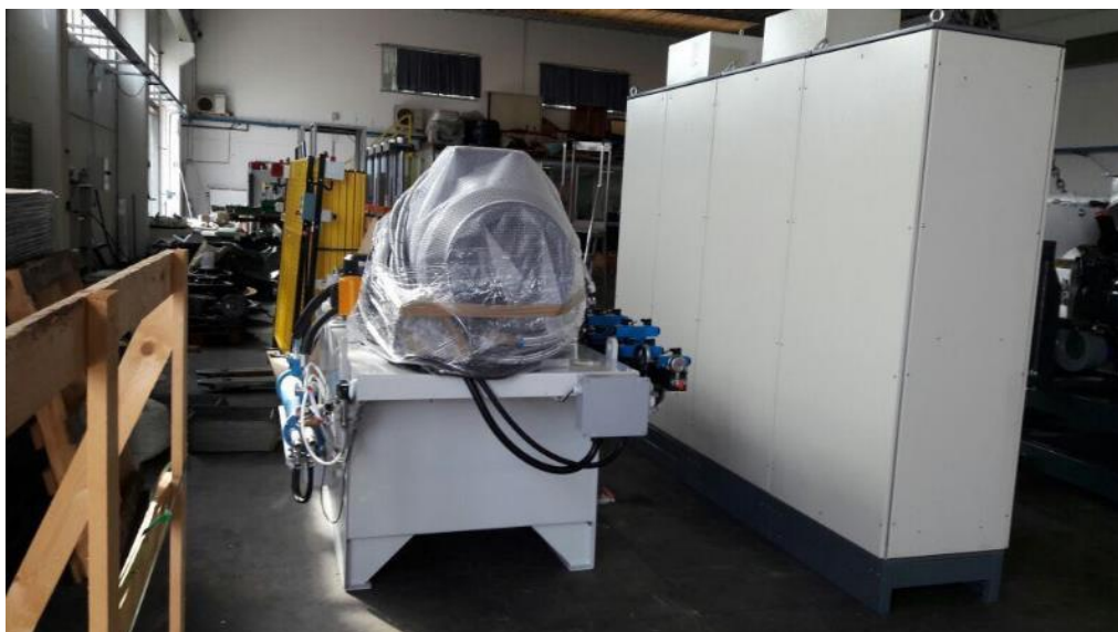
Installation of the injection unit at the demonstration site
